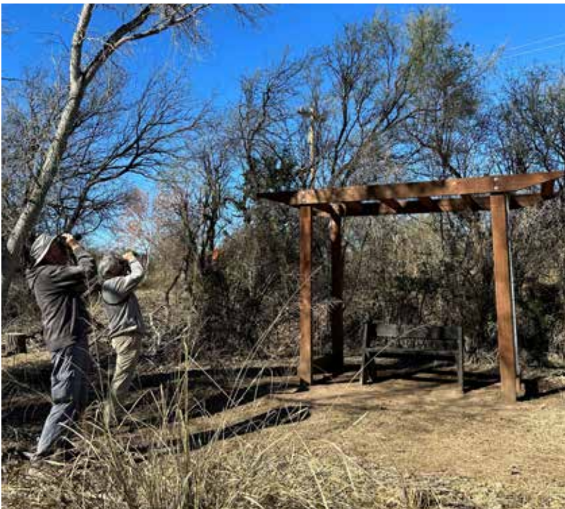
One of five new shade ramadas in the Cuckoo Corridor, Dan Lehman
