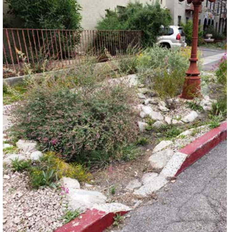
A basin awaits rainwater via a curb cut, Jennie MacFarland
